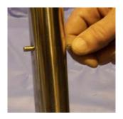
• To secure step, place one bolt (**D**) through the pre-drilled hole from the **outside** of the ladder and through the pre-drilled hole on the step.
